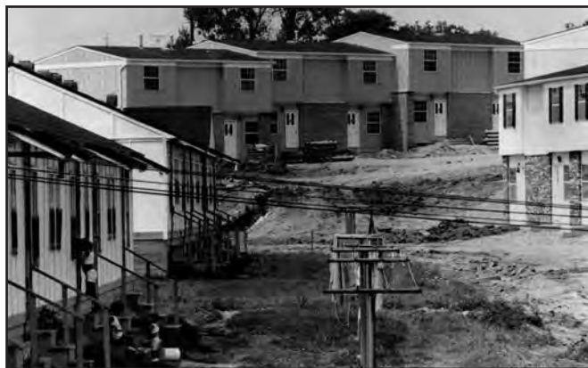
The “instant housing” units were constructed in Rochester, New York, and assembled on-site in Akron. While the process allowed AMHA to provide housing quickly, the construction methods did not hold up well over time, creating major maintenance problems.
