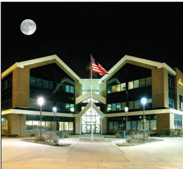
The central office building at 100 W. Cedar Street
