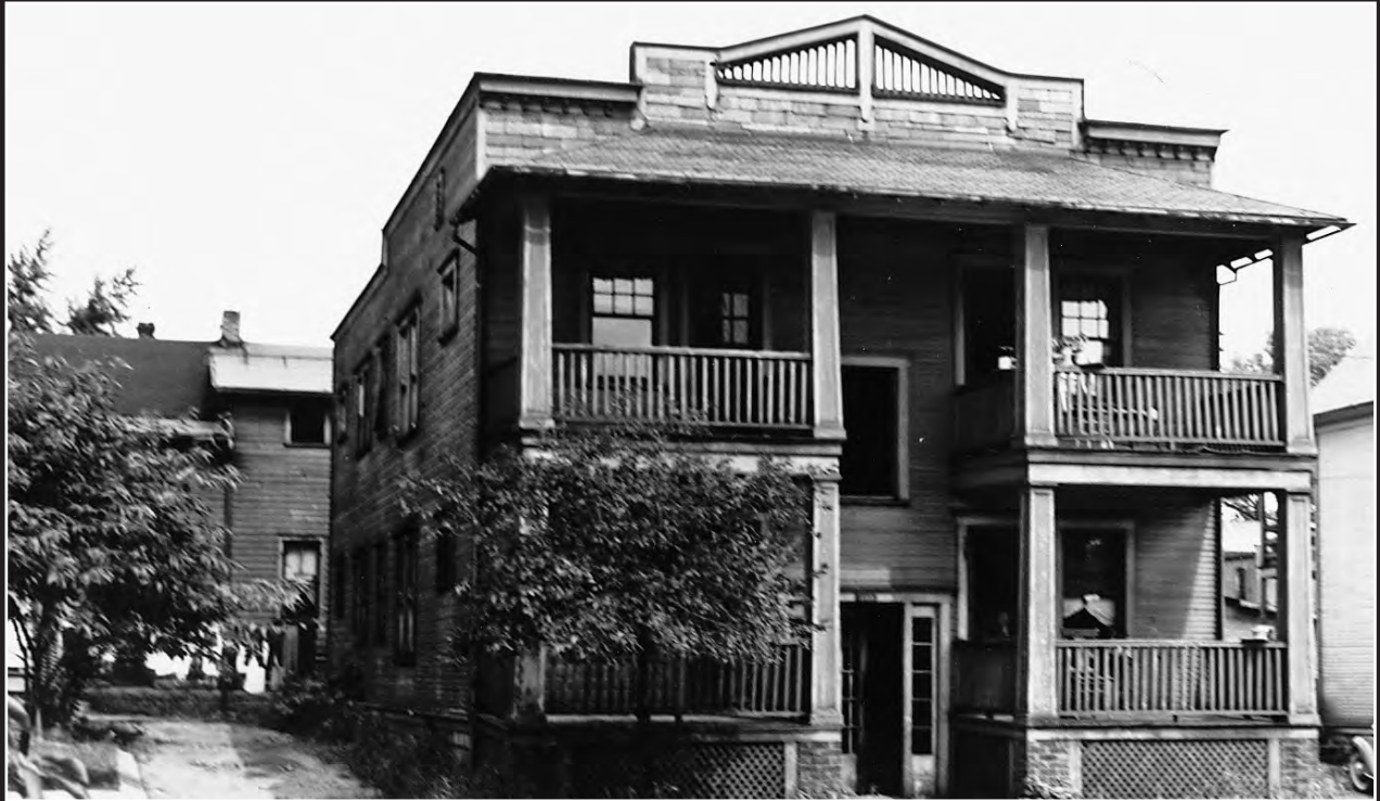
Akron, like most urban industrial areas, faced a critical shortage of housing during and after World War II. This property was typical of late 19th century construction showing a great deal of deterioration by the 1940s. This apartment building was demolished to make room for the construction of Edgewood Homes.
