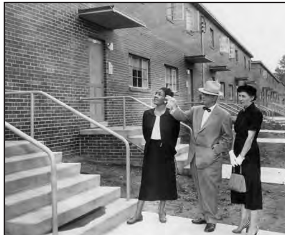
Additional housing was built at Elizabeth Park in 1956 to accommodate larger families. Inspecting the building is M. P. Lauer; his secretary, Mrs. Weyrick (right); and Elizabeth Park manager Wilhelmina Winston (left).
