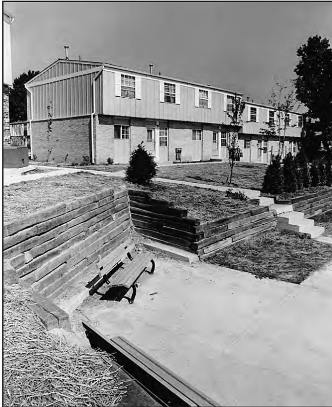
Construction of the Bon-Sue development on Biruta Street created some of the sharpest controversy Saferstein faced. West side residents protested, feeling that the public housing would adversely affect property values in their neighborhood.
